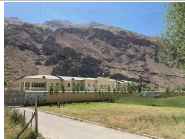
Photo 22: Mental hospital in Roshtkala district, upstream of reservoir
