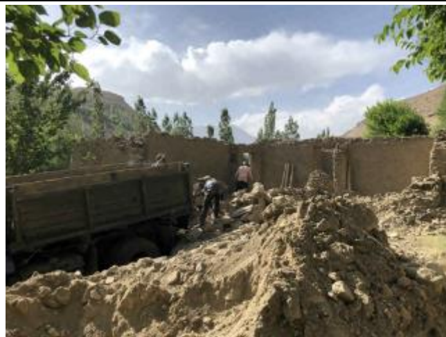
Photo 58: Demolishing of resettled family home at powerhouse
