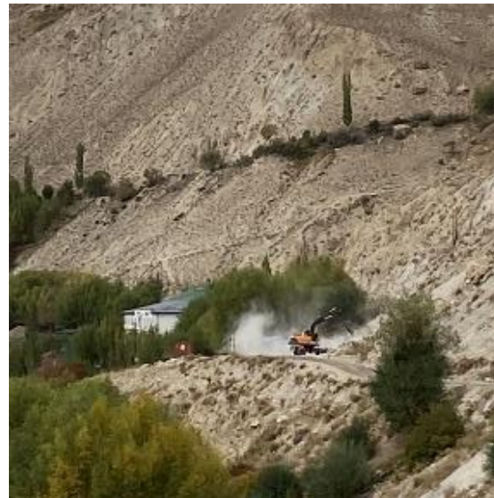
Photo 95: Dust plume generated by soil excavation near the base camp
