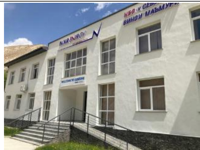
Photo 46: PEC Sebzor administrative building
