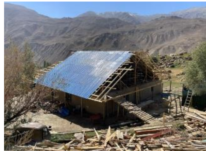
Photo 118: Nearly completed home at Upper Chagev
