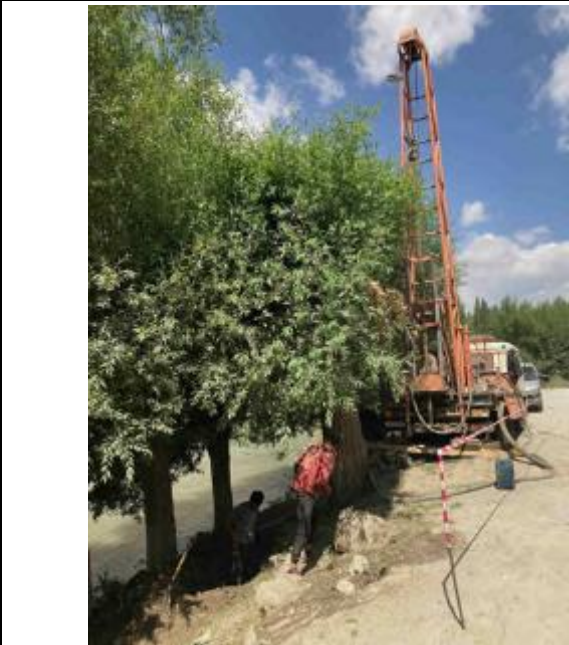
Photo 32: Test drilling at bridge upstream of intake
