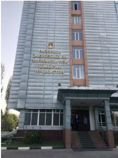
Photo 13: Ministry of Energy and Water Resources, Dushanbe
