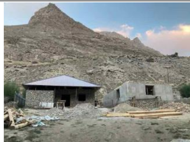
Photo 100: Replacement homes for homes destroyed in avalanche, funded by PEC and Ministry of Energy and Water Resources
