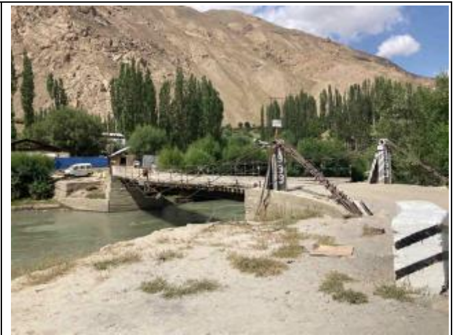
Photo 27: Old bridge upstream of intake
