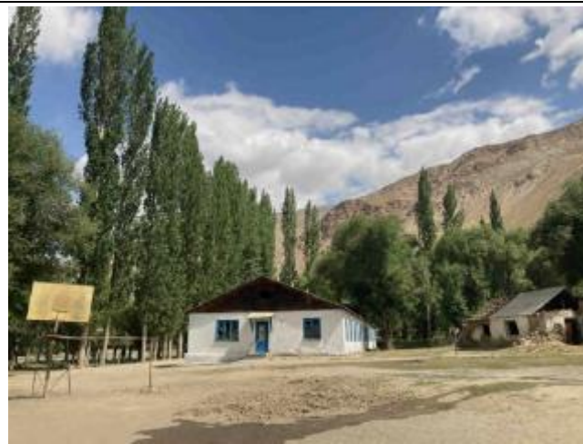
Photo 29: Old school on riverbank at reservoir
