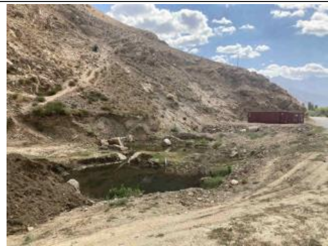
Photo 25: Spoil disposal area 1
