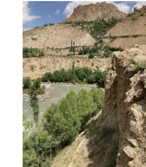
Photo 40: Steep riverbank at intake
