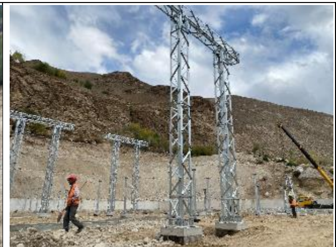
Photo 84: Sebzor substation under construction
