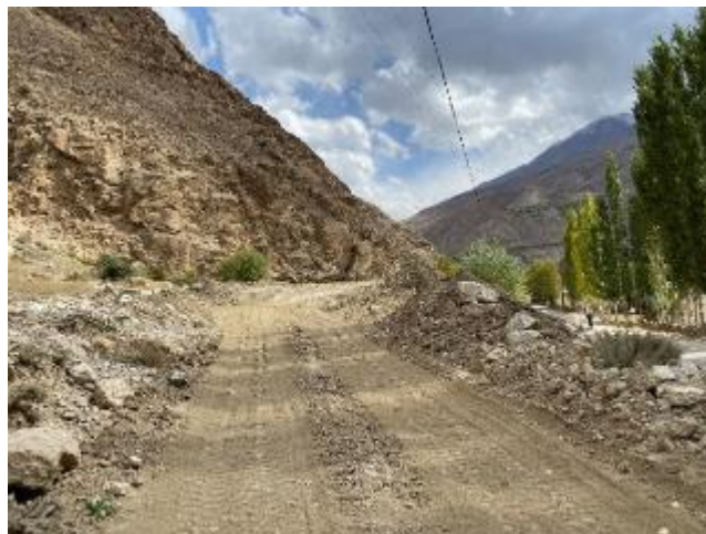
Photo 119: Temporary spoil and material storage area
