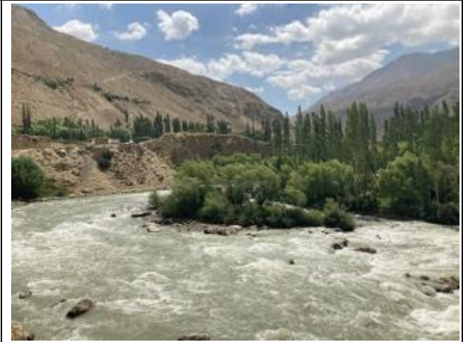
Photo 39: Intake area from downstream
