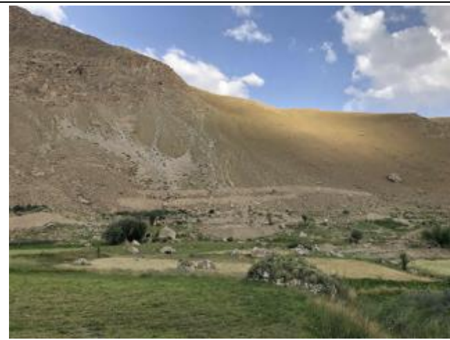
Photo 73: Terraces to protect Upper Chagev from rockfall
