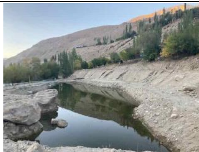
Photo 83: Excavation for Sebzor powerhouse
