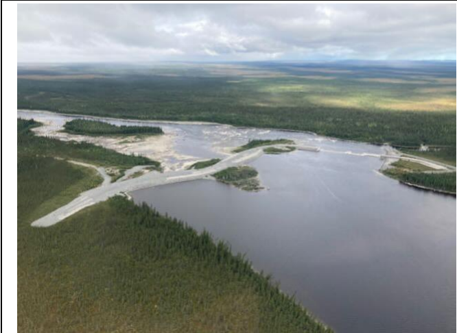
Photo 94: Rupert River weir
