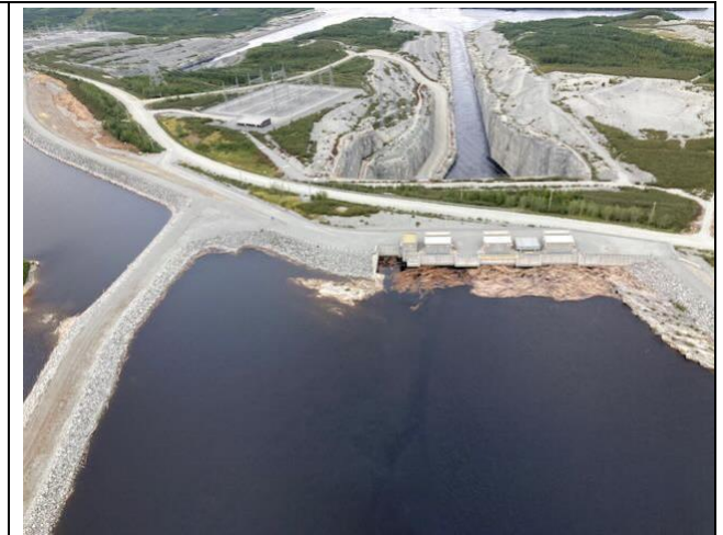
Photo 3: Eastmain-1a intake with floating logs
