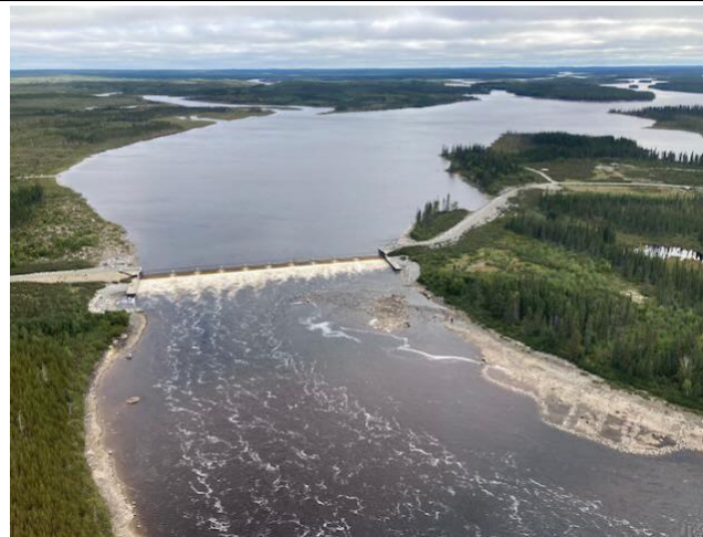
Photo 95: Rupert River weir with constructed spawning sites
