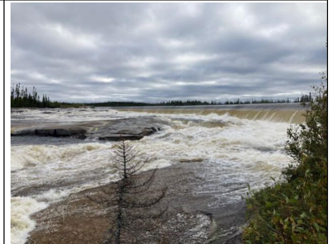
Photo 102: Weir from downstream
