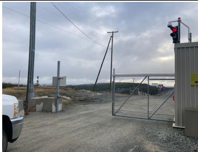
Photo 41: Entrance controls at Eastmain dam
