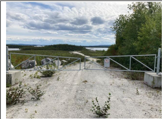
Photo 73: Access road to Rupert forebay near Tommy Neeposh Tunnel
