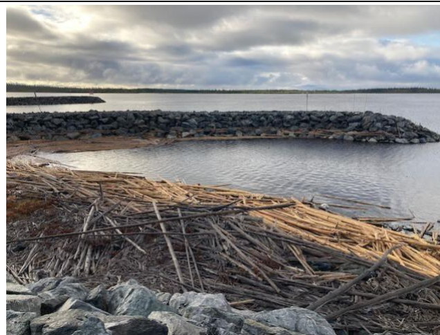
Photo 44: Debris and warning signs in front of Eastmain spillway
