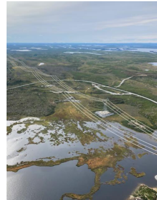
Photo 72: Transmission lines crossing Rupert tailbay
