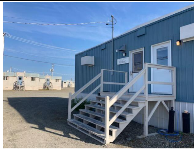
Photo 20: Elevated office entrances for snow conditions
