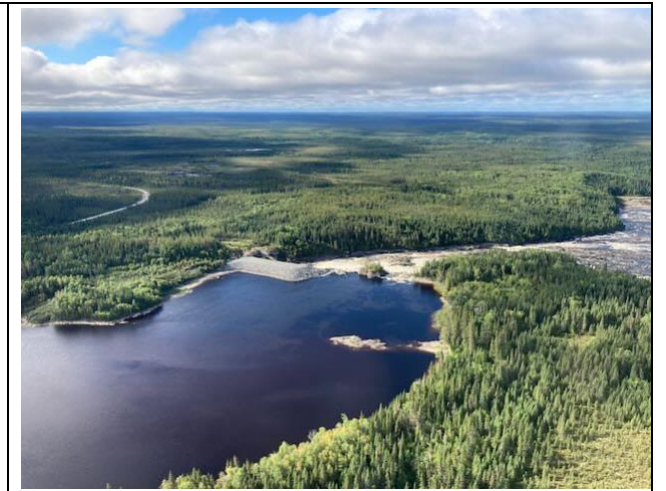
Photo 93: Rupert River weir
