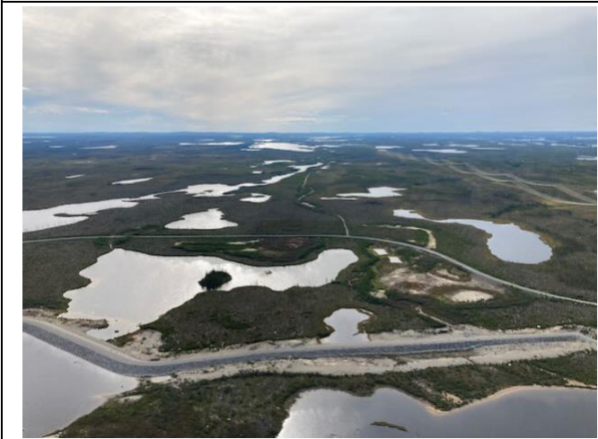
Photo 76: Embankment dikes on Rupert tailbay
