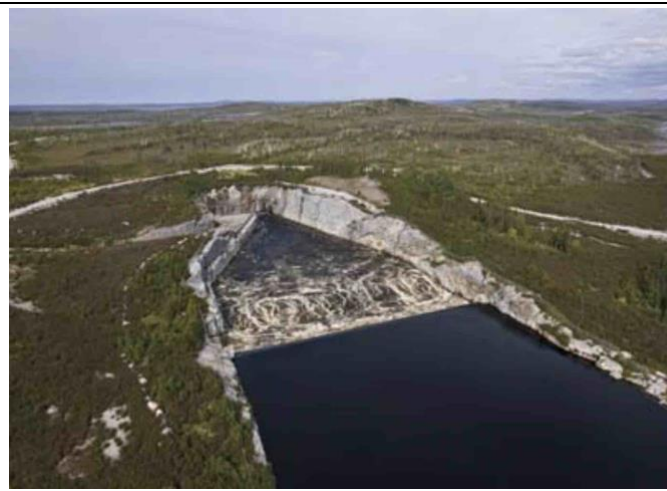
Photo 74: Tommy Neeposh Tunnel intake
