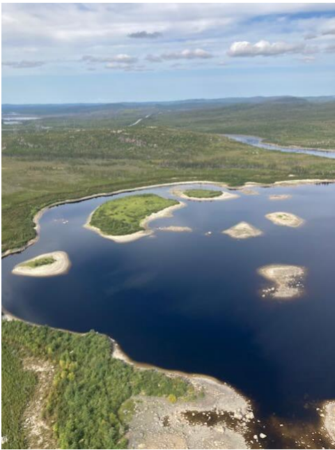
Photo 106: Bay below Rupert diversion dam
