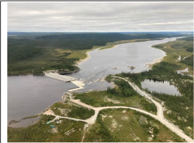
Photo 91: Rupert River weir
