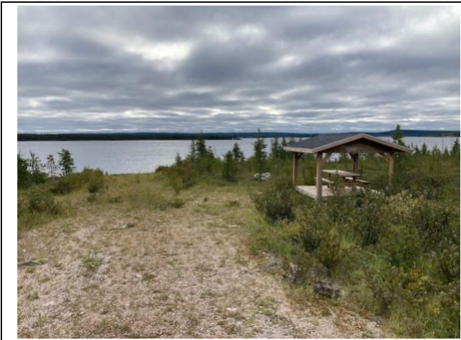
Photo 97: Boat ramp with shelter above weir
