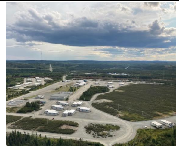
Photo 18: Camp with rehabilitated part on right
