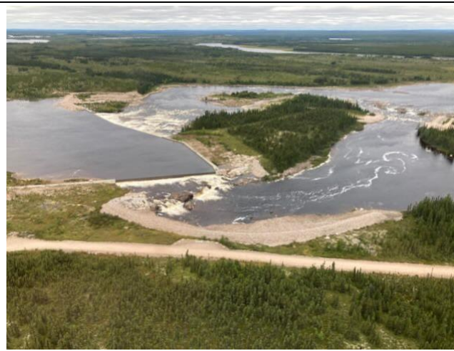
Photo 92: Rupert River weir
