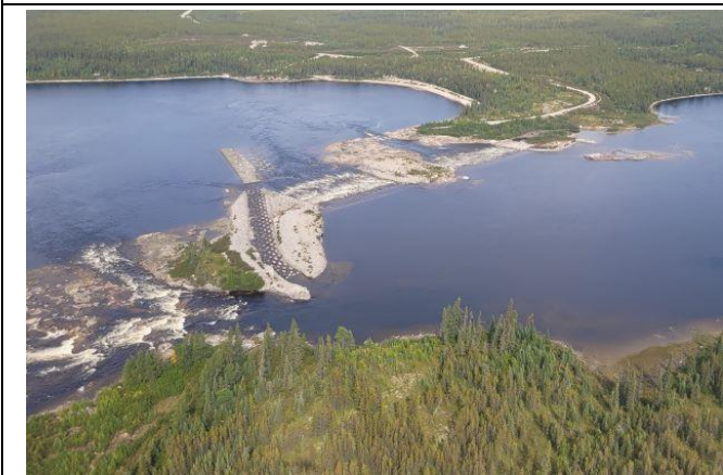
Photo 136: Fish passage on Rupert River
