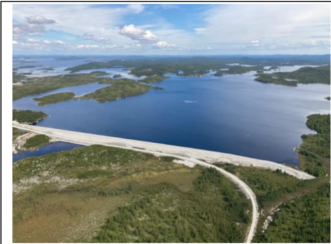
Photo 67: Rupert diversion dam and forebay
