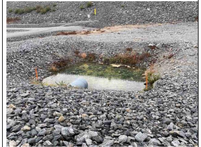
Photo 54: Seepage monitoring below Eastmain dam
