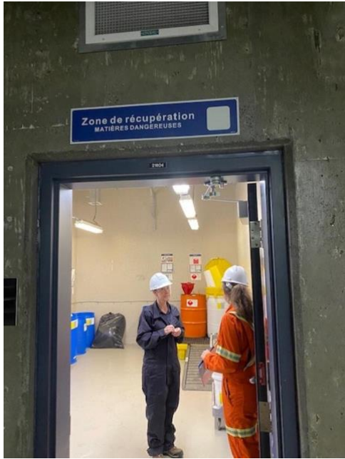
Photo 7: Waste separation room
