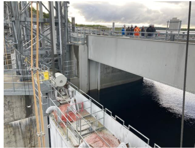
Photo 53: Eastmain dam spillway gates
