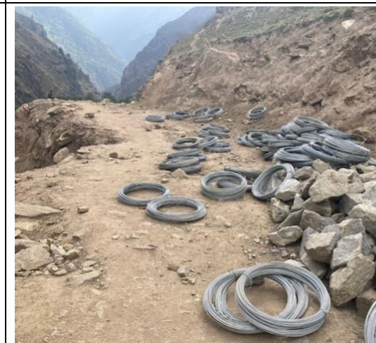
Photo 30: Material to build gabions for road improvements
