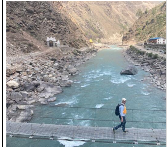
Photo 48: Bridge just upstream of Kharpunath temple
