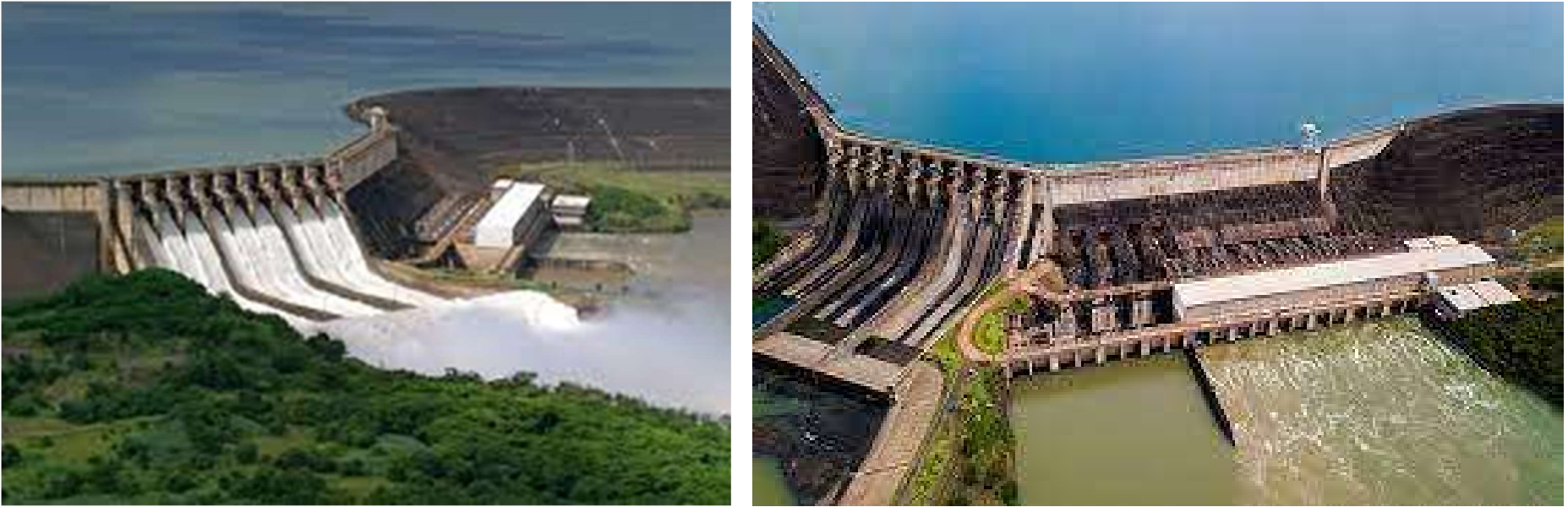
Figure 2 – Aerial views of the São Simão HPP: during a period of high flow (on the right) with all 9 spillway gates open, the flip bucket/ski jump dissipator discharging flows downstream in the Paranaíba River, and left: view of the tailrace area where flow is being discharged downstream.
