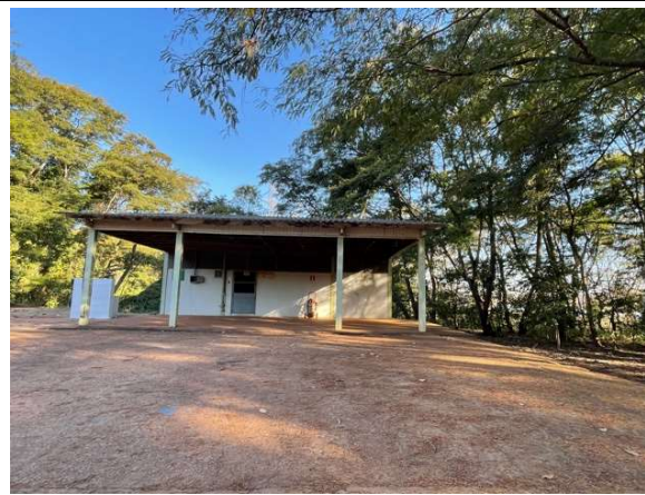
Photo 10: São Simão HPP hazardous waste deposit
