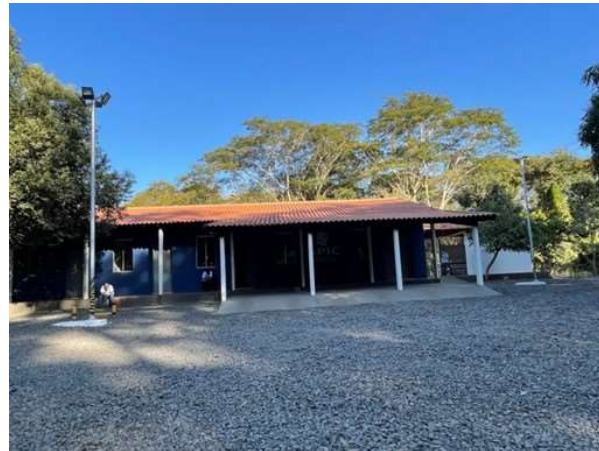
Photo 34: SPIC Modernization Project Headquarters Offices at the powerplant
