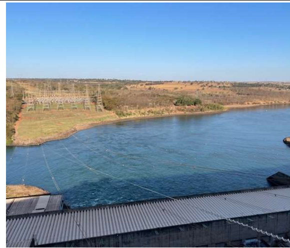
Photo 18: Transmission line from São Simão powerhouse to CTEEP Substation
