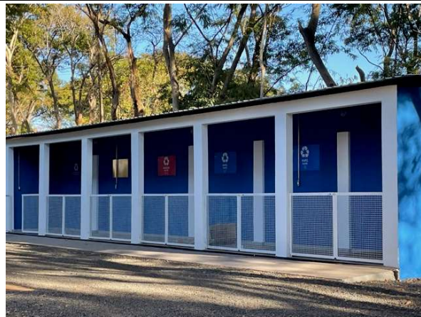
Photo 9: São Simão HPP central recycling Unit
