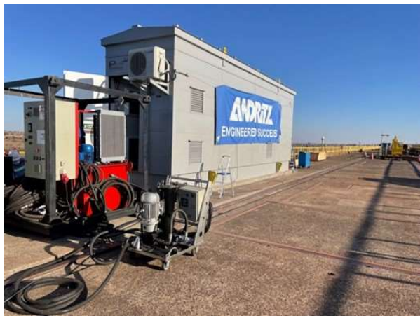
Photo 33: Modernization Project activities at dam crest
