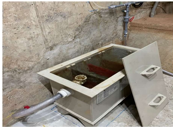
Photo 21: Biobox that monitors the Golden mussel's presence and residual chlorine levels in the water
