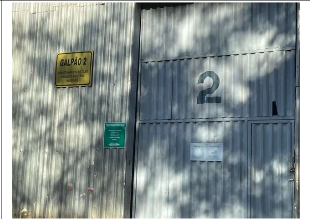
Photo 11: Oil, fuel, non-hazardous residue and scrap deposit
