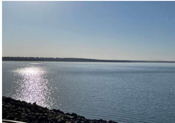
Photo 22: Right bank of the reservoir upstream view from the dam crest
