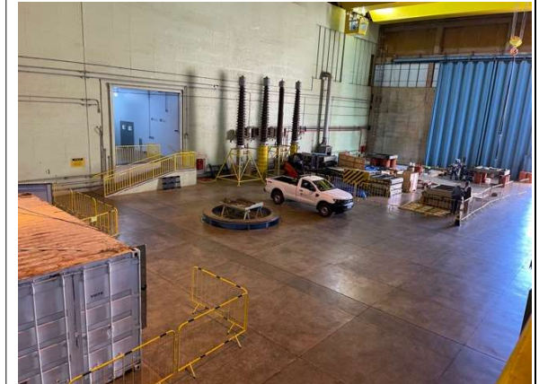
Photo 32: Powerplant Modernization Project Contractor's activities inside the powerhouse
