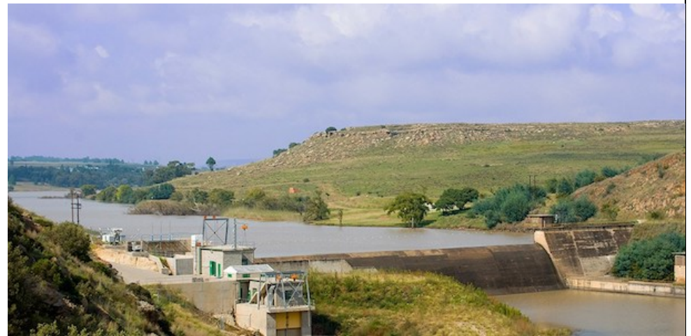
Photo 7: Operational Sol Plaatje hydropower project, next to Sol Plaatje dam ( https://www.rehgroup.co.za/project/sol-plaatje/ )
