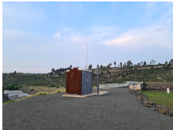
Photo 4: Intake gate structure with view to right bank
