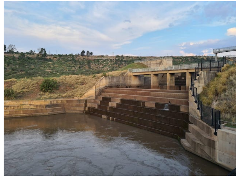
Photo 9: Spillway from downstream, with tailrace in foreground
