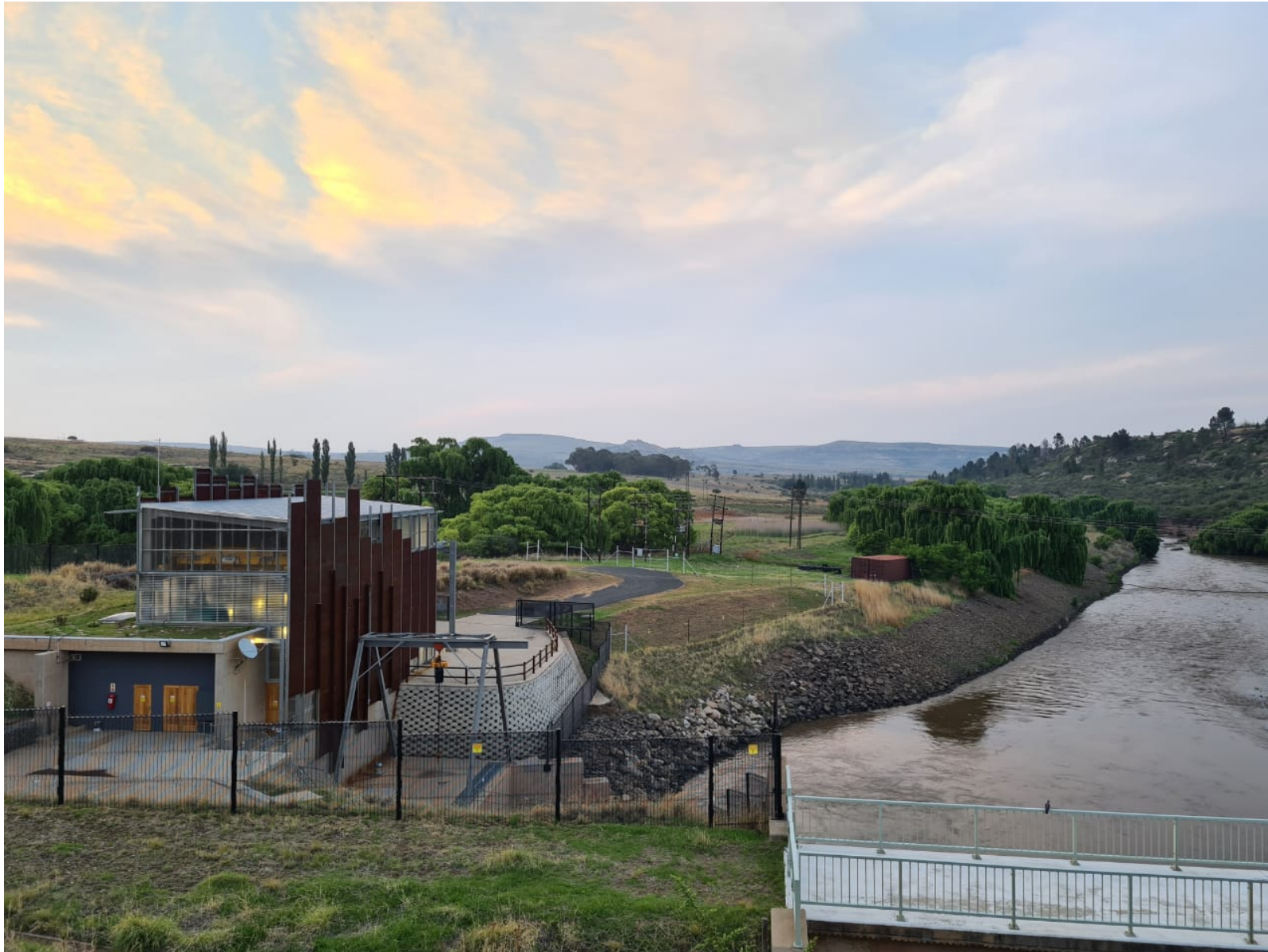
Figure 1 – View from the Botterkloof Dam, with the Stortemelk powerhouse on the left and the Ash River flowing downstream. Note the architecturally distinct design of the powerhouse, the fencing around REH's property, the small storage building to the right, riprap for erosion protection along the riverbanks, the successful revegetation of the construction site, and the wetland on the left bank.
