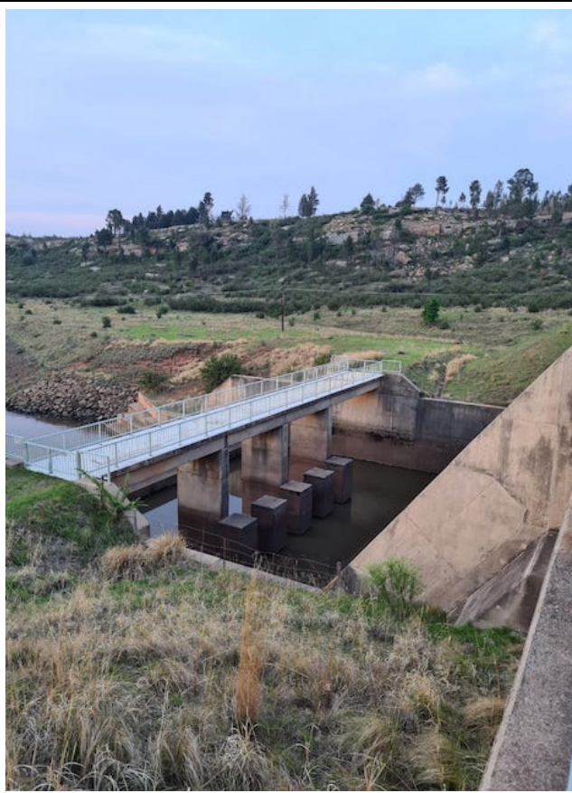
Photo 6: Spillway from upstream, with energy dissipators
