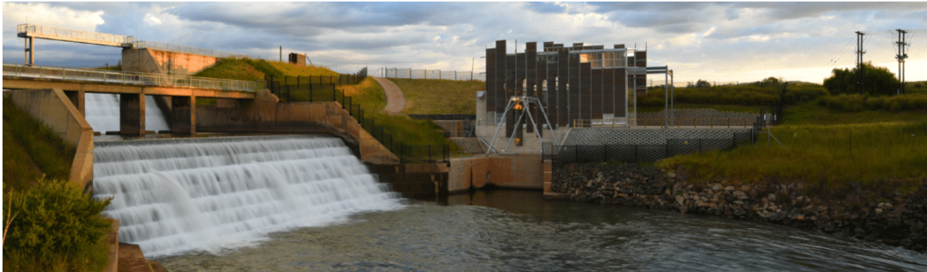
Photo 3: View of Botterkloof spillway, Stortemelk power station and transmission line from right bank ( https://www.zutari.com/project/stortemelk-hydropower/ )
