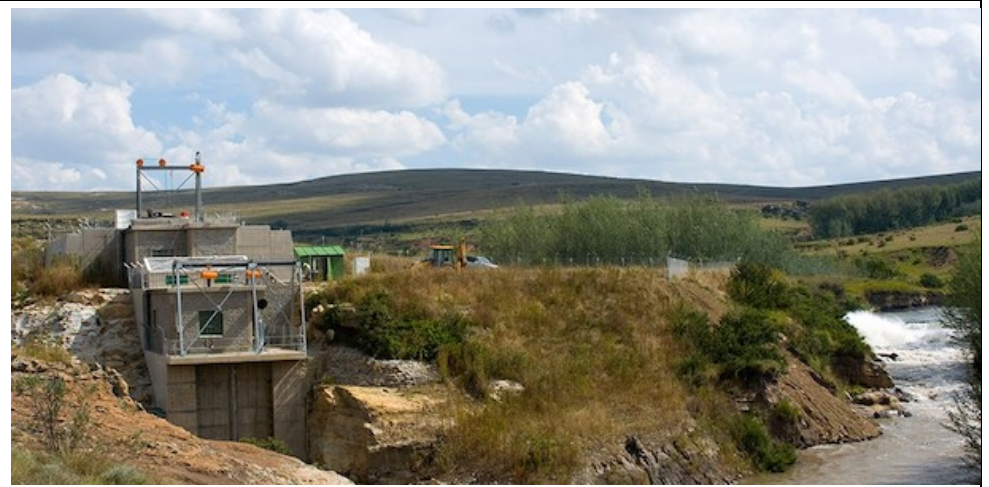
Photo 5: Operational Merino hydropower project ( https://www.rehgroup.co.za/project/merino/ )
