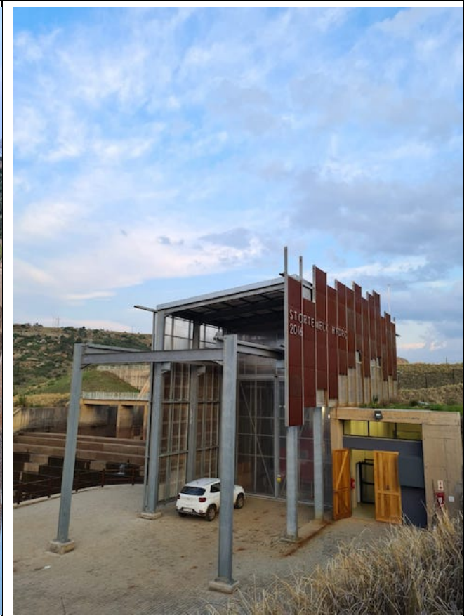
Photo 7: Powerhouse from northwest, with generator on left and transformer on right
