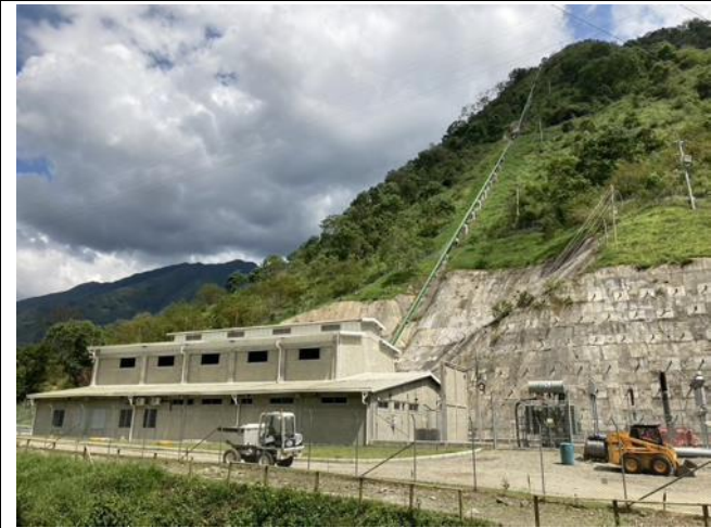
Photo 16: La Chorrera penstock and powerhouse
