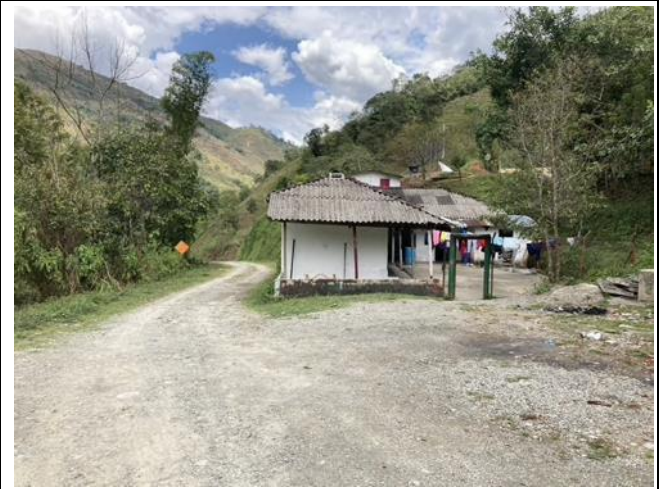
Photo 15: Junction of 25AN with access road to La Chorrera powerhouse, upstream of Chorreritas
