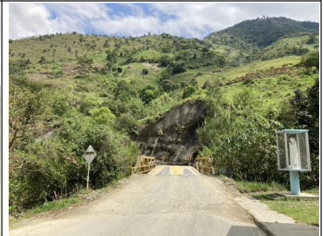
Photo 12: 25AN road bridge over San Andrés River at Alto Seco
