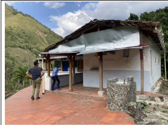
Photo 28: Acquired house above future bridges
