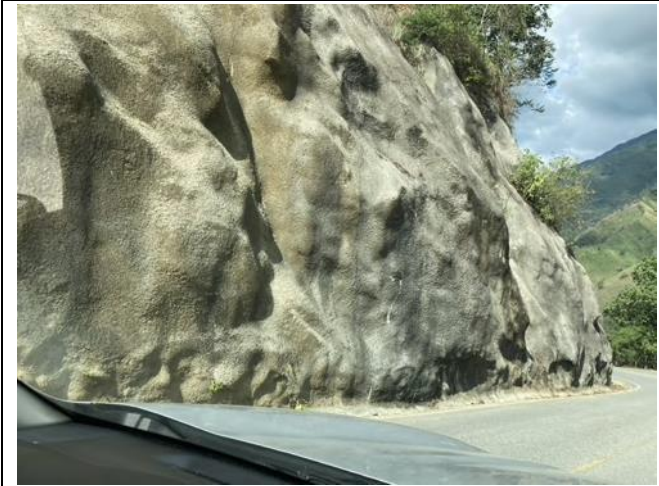
Photo 34: Slope above future tunnel entrance on left bank
