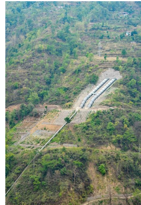
Photo 18: The surge shaft and the bioengineering done there to control erosion.
