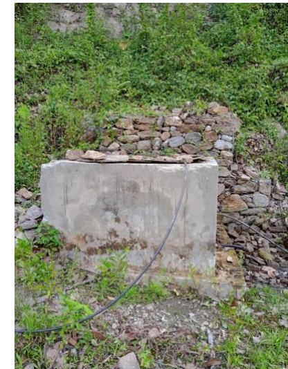
Photo 42: Safe drinking water provided at the cremation place built as a community benefit.
