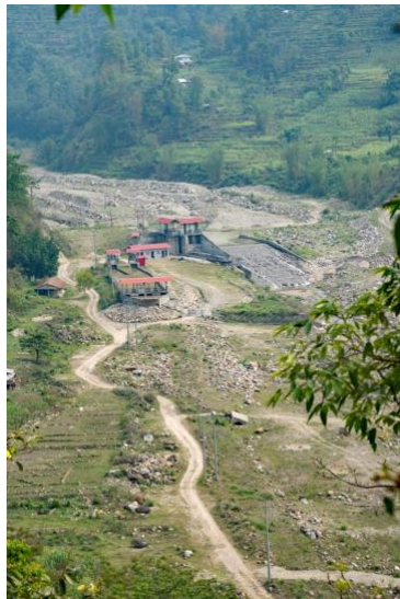
Photo 1: The Mai Beni HPP weir, intake and desander, with cremation-site shelter at centre-left.
