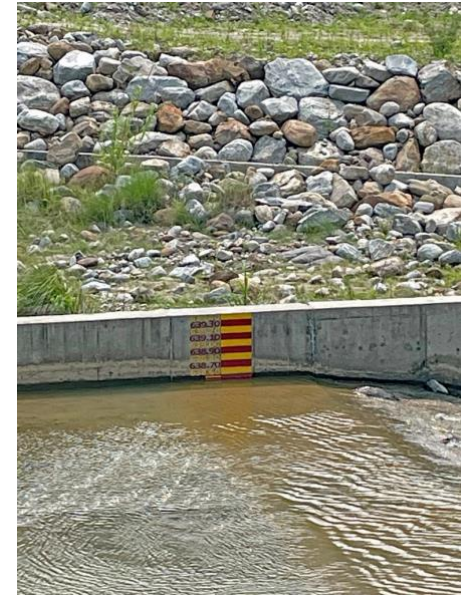
Photo 51: Discharge gauge for monitoring of environmental -flow releases at the Mai Beni weir.
