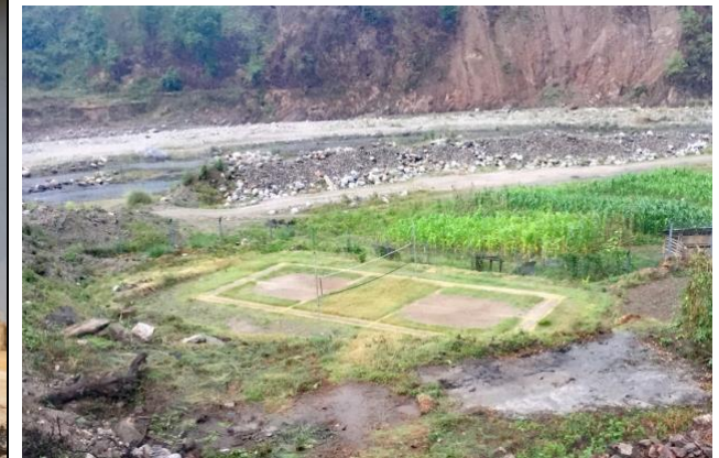
Photo 12: Badminton court for Mai Beni staff, note severe bank erosion, caused by normal flood flows, in the background.
