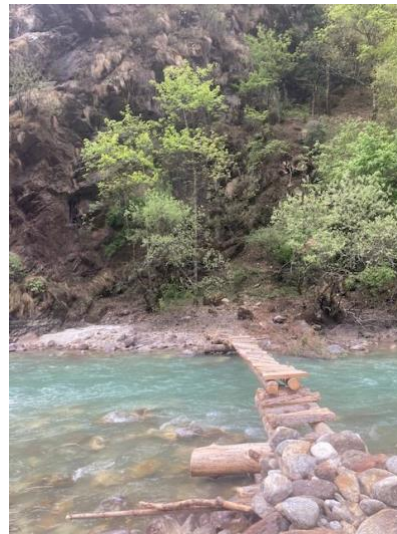
Photo 5: Bridge for flow measurements at headpond area
