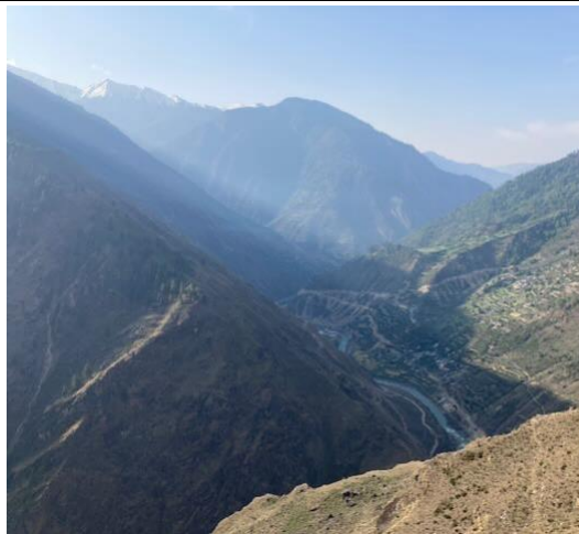
Photo 52: View into Karnali valley downstream of Chuwa confluence and Kharpunath village
