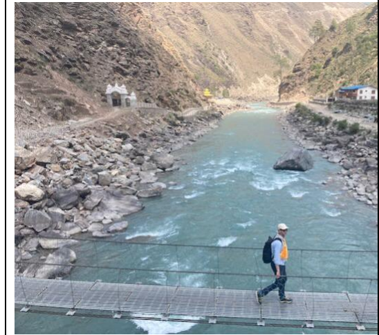
Photo 48: Bridge just upstream of Kharpunath temple
