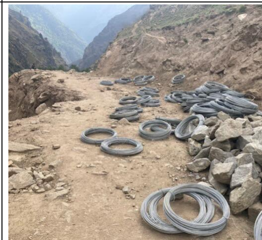
Photo 30: Material to build gabions for road improvements
